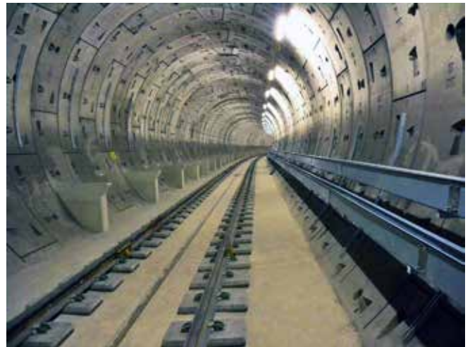
Canal tunnel shortly after track laying
